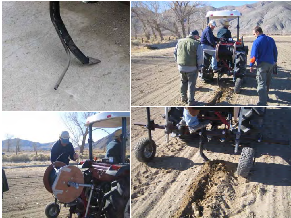
Figure 7. Installation of fiber optic cable at the Valley Vista ranch site in December 2007. Approximately 1,000 m of fiber was installed at both Alternative Agriculture sites.
