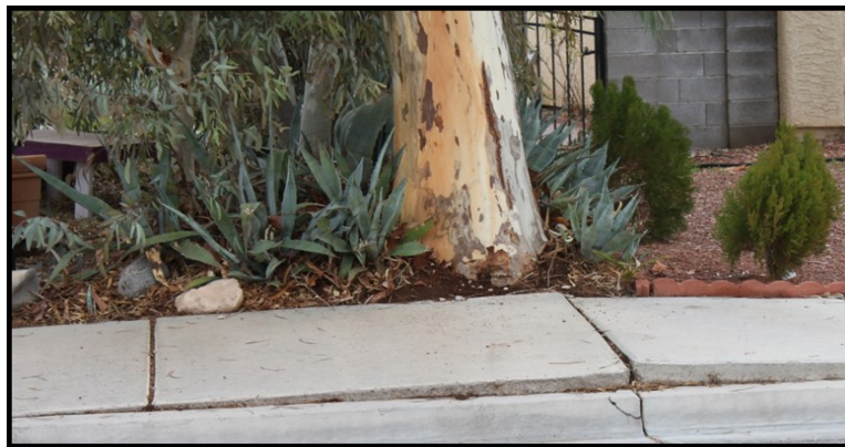
Figure 7. Here is a large Eucalyptus root lifting the sidewalk. When sidewalks are lifted like this, they are a hazard to pedestrians.
